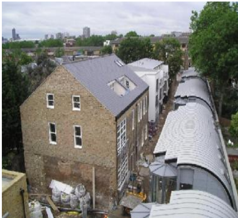
Aerial View of Clare Lane
