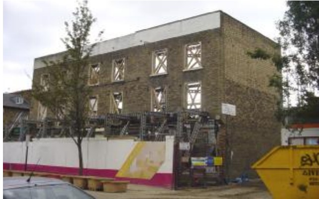
Halliford Street: Retained Facade and Flank Walls
