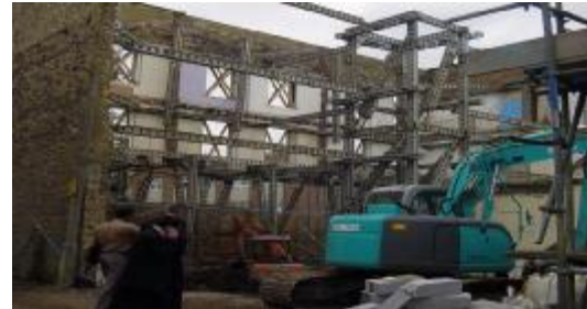
Halliford Street: Facade Retention Framework
