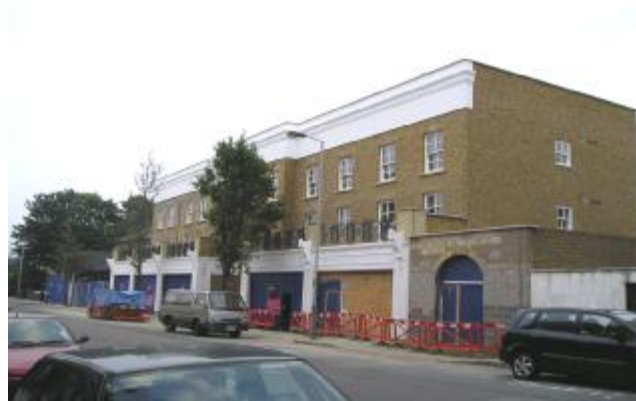
Halliford Street: Retained and Extended Facade
