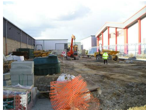
Infrastructure Works to the Rear of the Site
